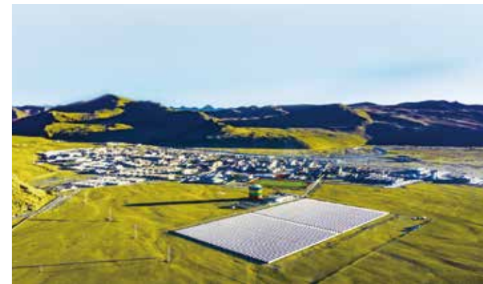
PV+Solar Thermal+Energy Storage Project, Tibet
